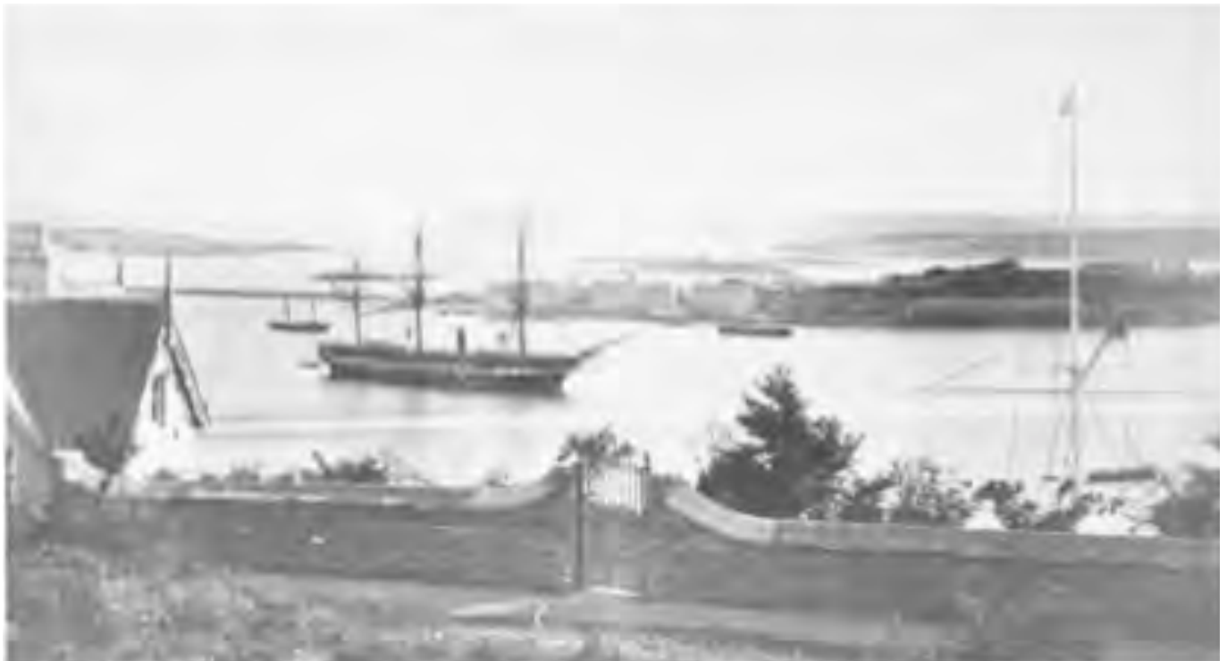
Queenstown (Cobh) in 1868
